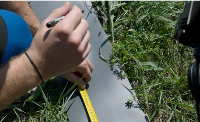
1 Unroll the shade fence filling and cut it to the width of the mesh.
