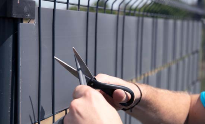
5 The form of the fence filling can be easily adjusted by cutting it.
