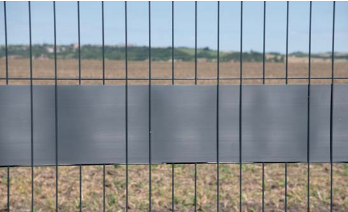
3 Weave from the first row along the entire length of the fence, ideally two meshes at a time.
