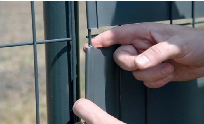
4 Secure the ends of the filling around the last pole with the clips provided.
