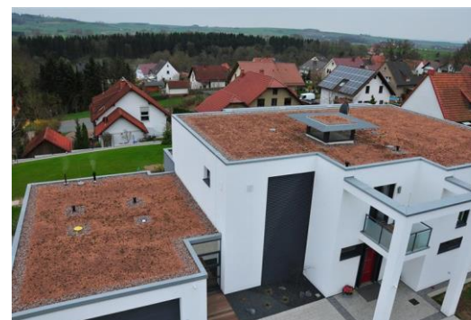
FIGURE 6: SHOWS THE MAPEPLAN T INSTALLED ON GREEN ROOF WITH SOIL BALLAST
