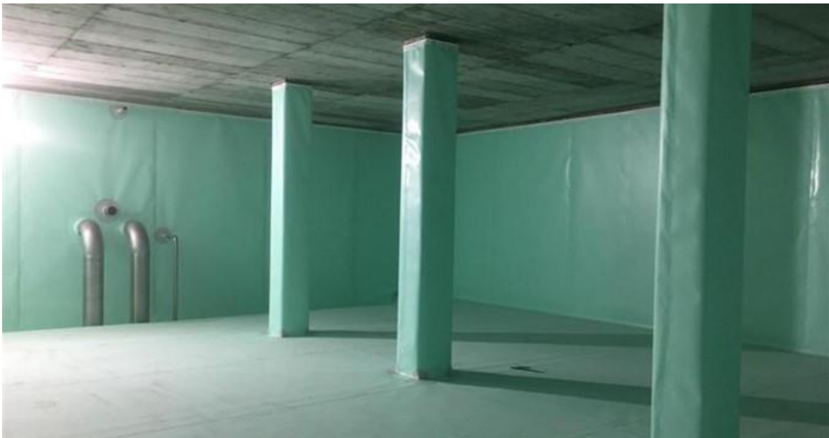
Figure 8: Installation of Membrane MAPEPLAN T WT on a water tank
