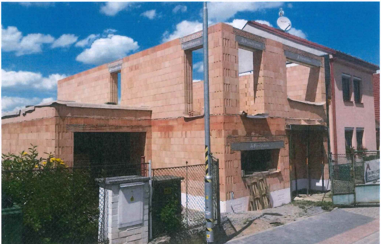
Photo 6 – Built-in KP Vario UNI lintels
