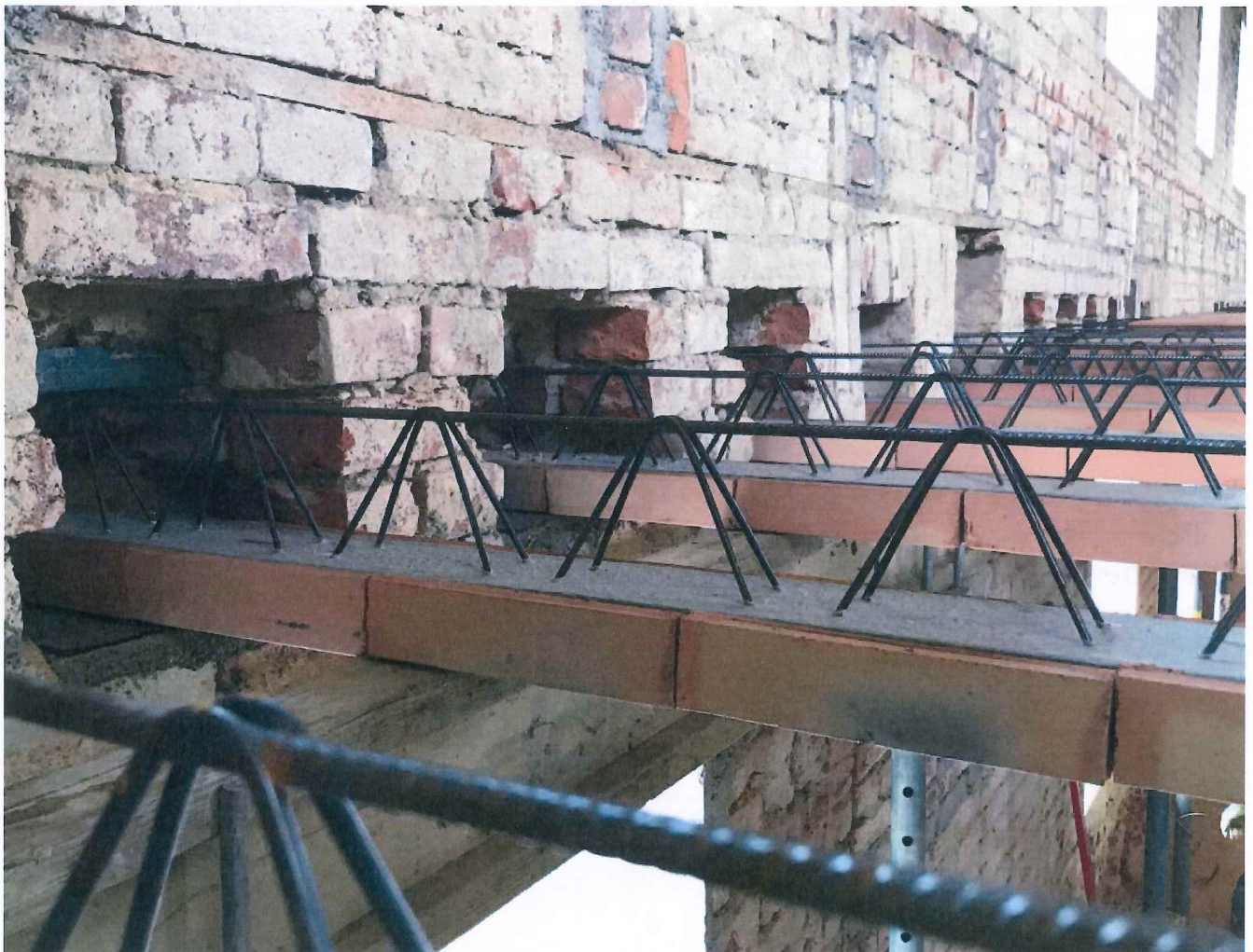
Photo 8 – Ceiling beams POT used for building reconstruction
