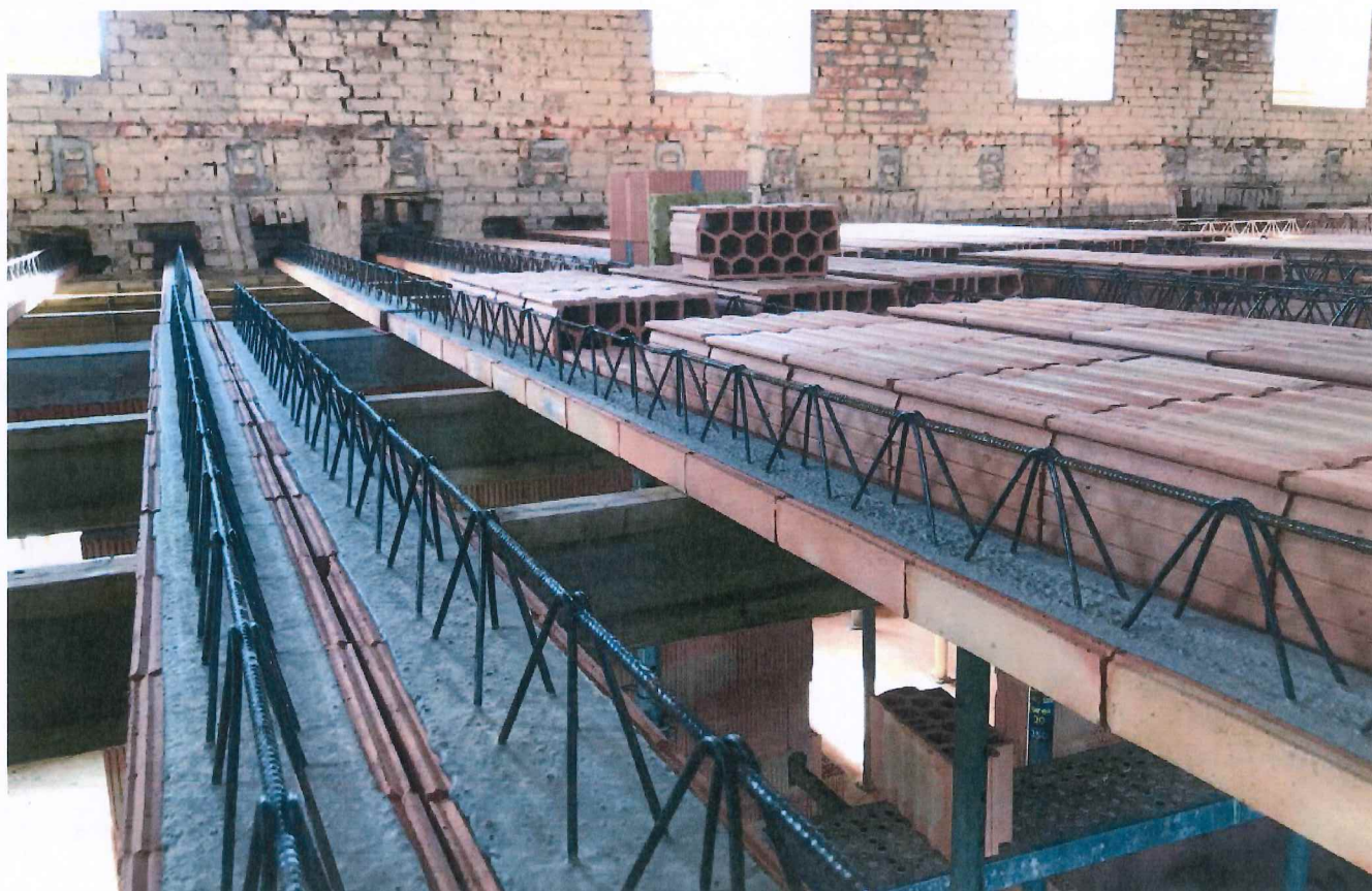
Photo 7 – Ceiling beams POT used for building reconstruction
