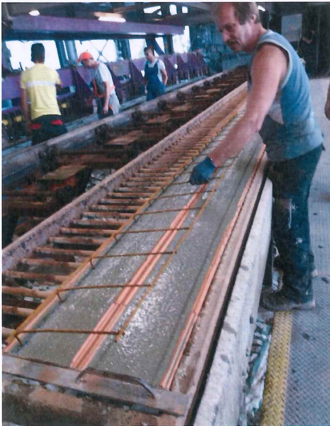
Photo 4 – Inserting steel reinforcement
