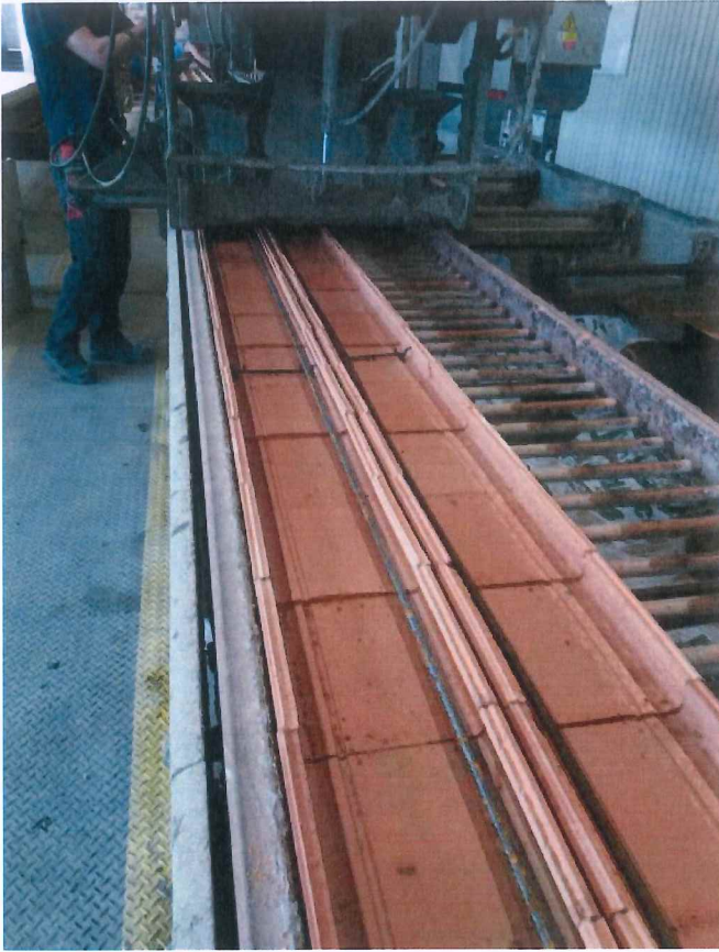
Photo 2 – Moistured U-shaped masonry units before concrete placement
