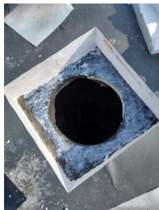
Krok 2 – penetrace hydroizolace
