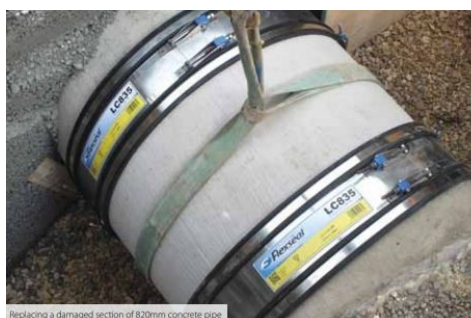
Replacing a damaged section of 820mm concrete pipe
